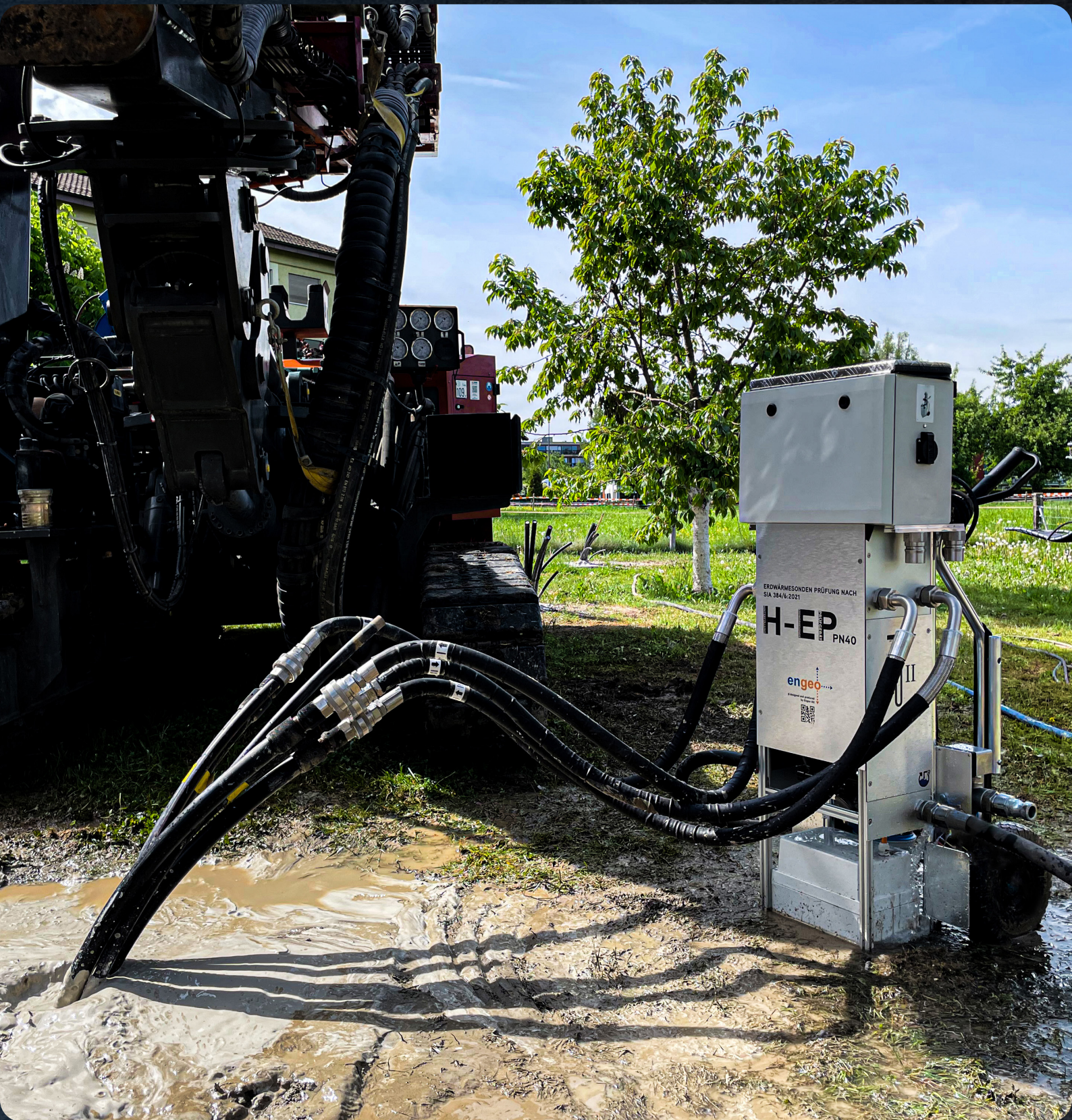
HEP during geothermal BHE testing
